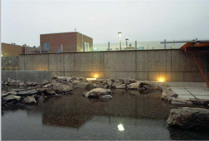
Side view of the ACTIFLO basins
