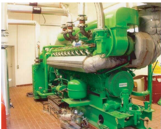
1.0- MW Gas Engine Supplying Heat for BioCon Dryer
