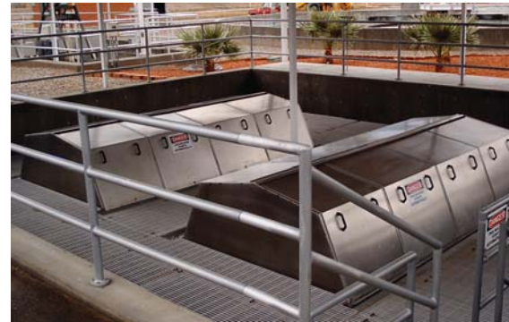
Hydrotech Discfilter Installation Mesquite, NV
