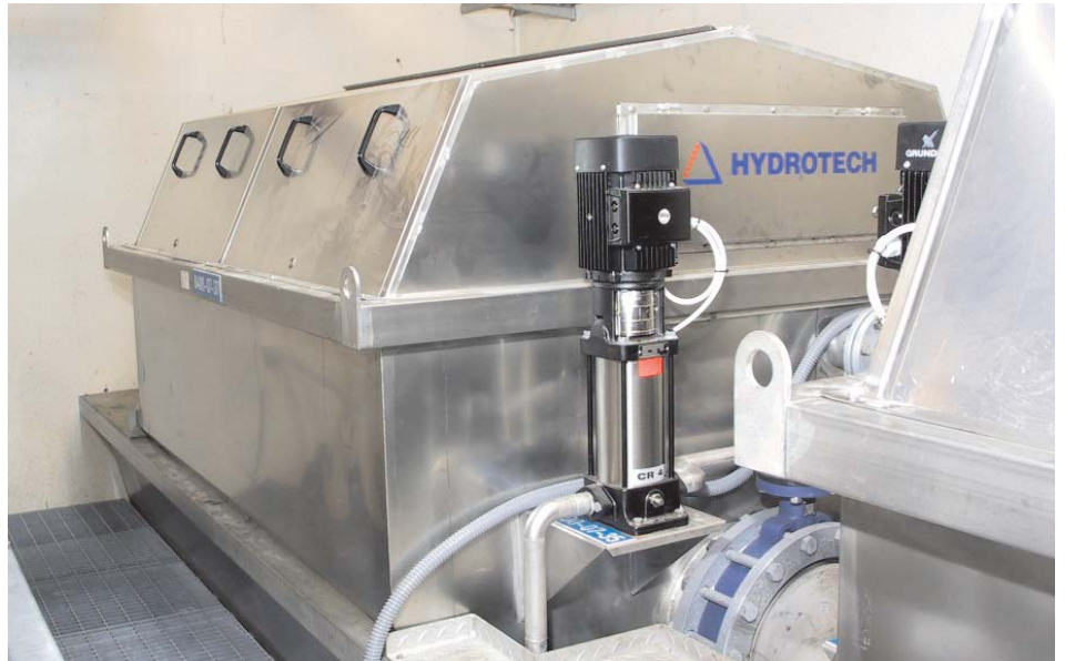
Rinse water pump arrangement
