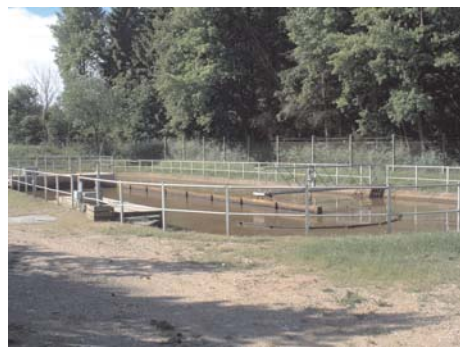
Picture: Sdr Vissing wwtp in Denmark.
