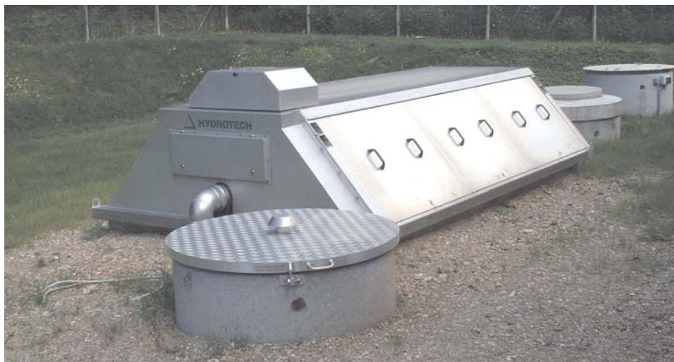
Picture: Hydrotech Drumfilter HDF2007-1L, 18 µm filter opening, maximum flow 50 l/s.
