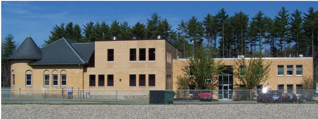
The City of Somersworth Plant
