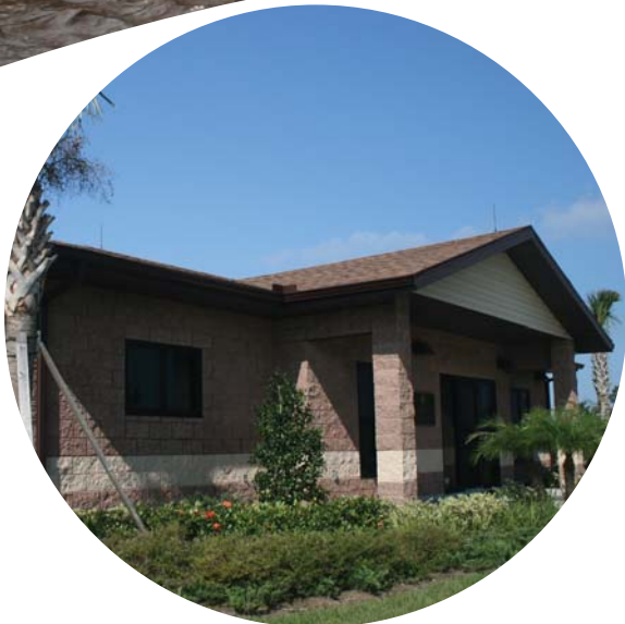
Sanford South Water Resource Center
