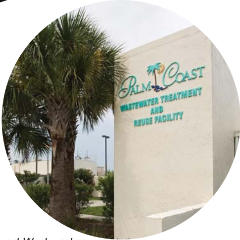
Palm Coast Wastewater Treatment and Reuse Facility
