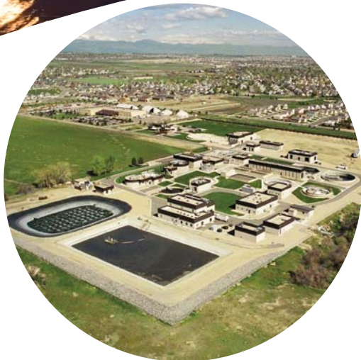
Aerial of Broomfield, CO WWTP
